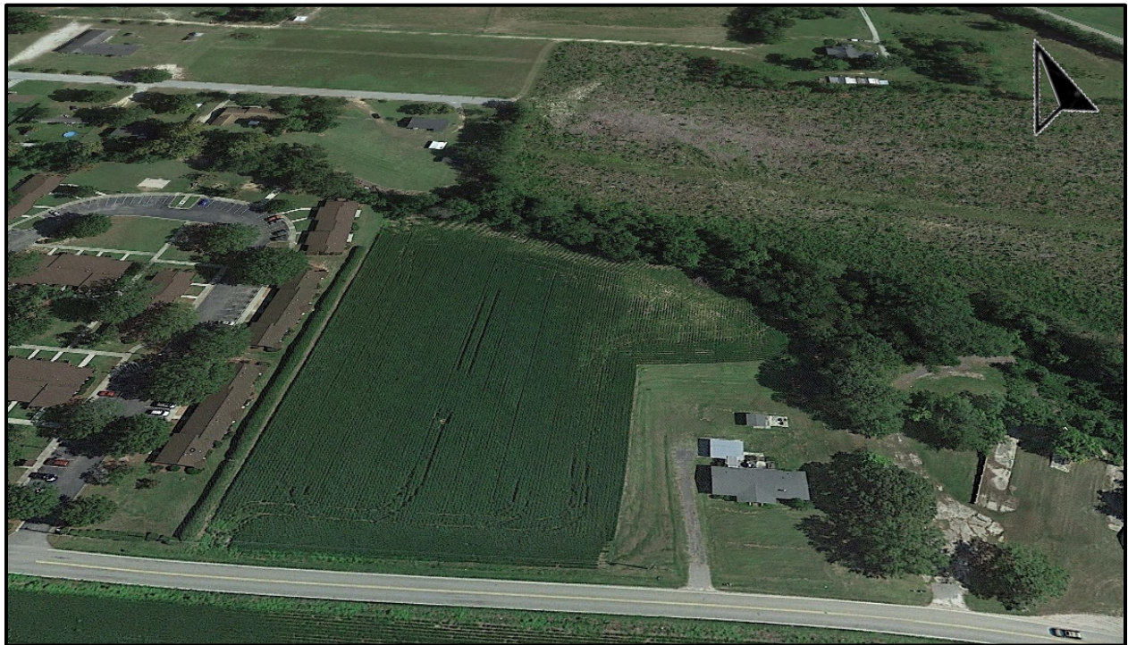
EXHIBIT 4. ACADEMY ROAD EXISTING CONDITIONS LOOKING NORTHEAST
